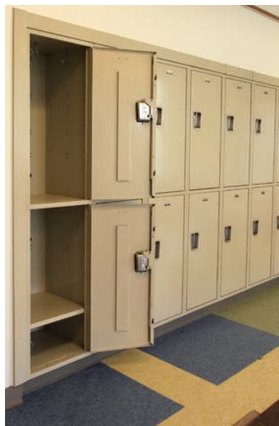
ADA locker has shelf at least 15 inches from floor.
